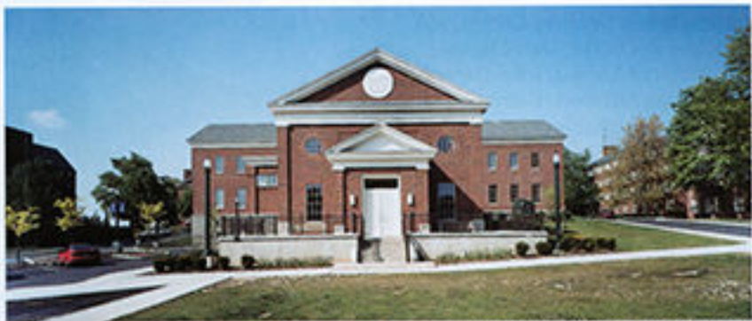
Entrance to recital hall lobby
